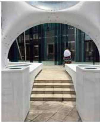
A- FIBER GLASS & METAL STUDS
