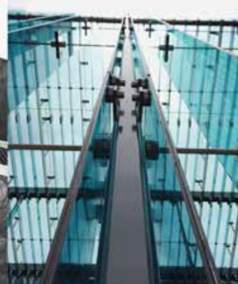
F- TINTED GLASS, CABLES AND METAL STUDS
